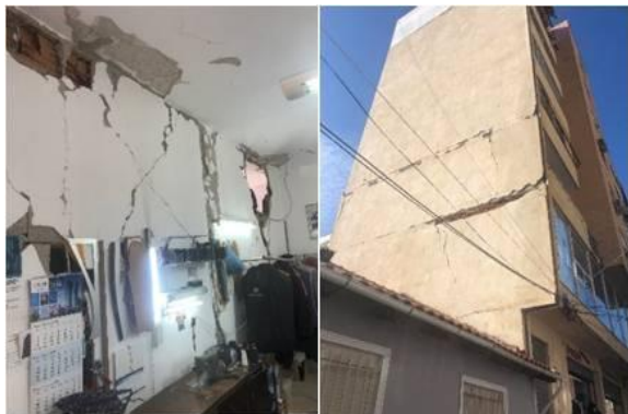
Fig. 5 Damages of non-structural elements.
